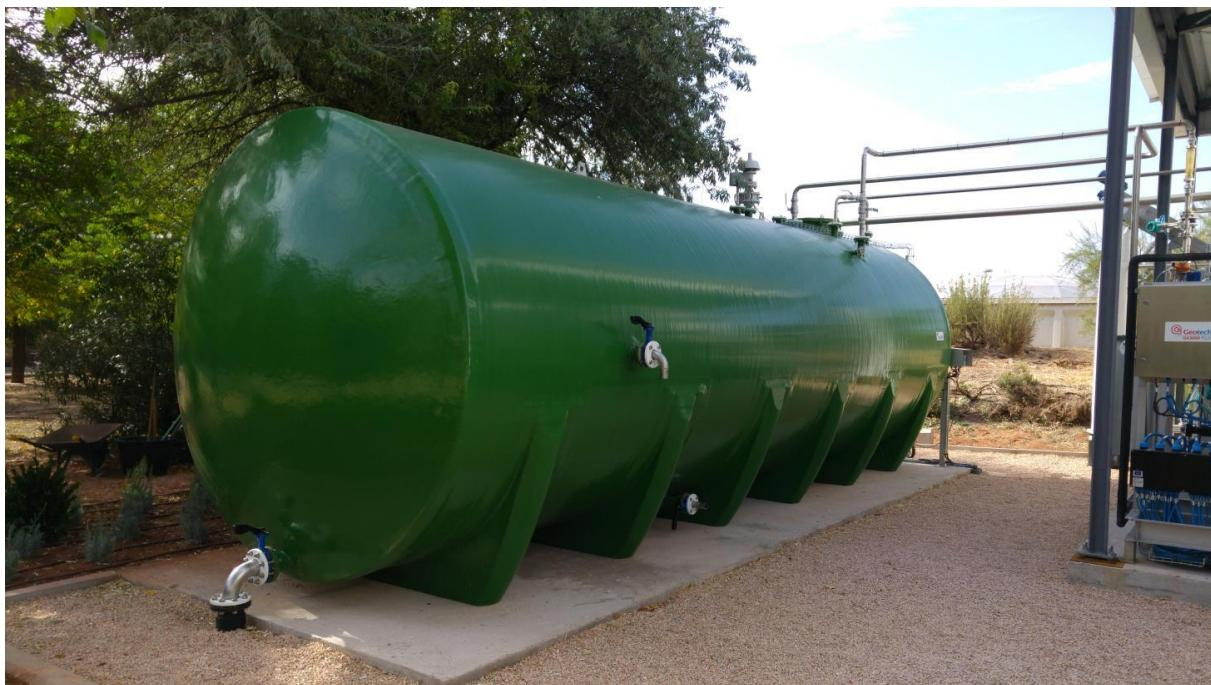
**Figure 4: Anaerobic Reactor (40 m<sup>3</sup>)**
