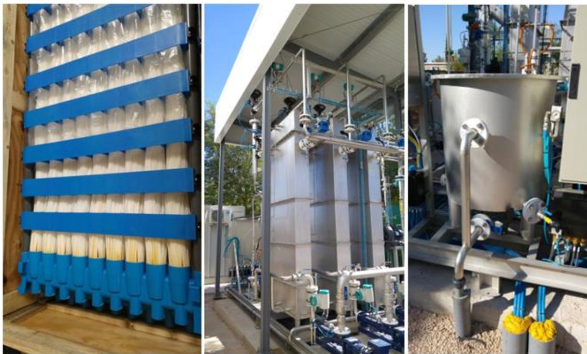
**Figure 5: 3 Membrane tanks (PURON®, KMS, 41 m<sup>2</sup> filtration area/module, Ultrafiltration (0.03 µm)) and CIP tank**
